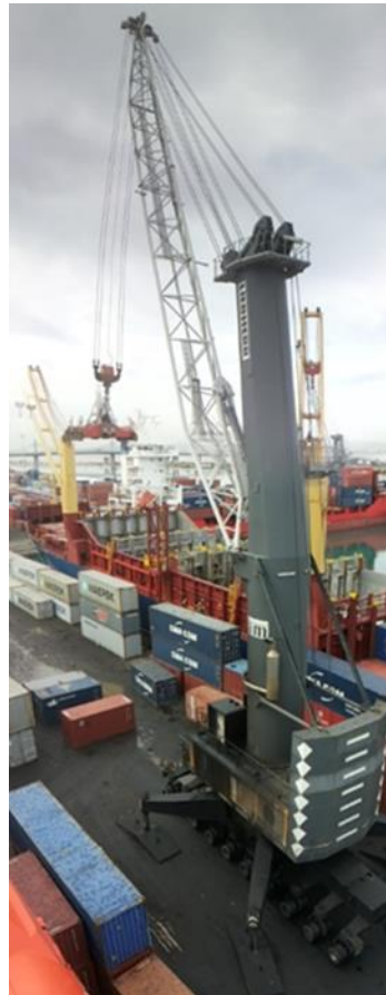
Fig. 5. Mobile shore crane
