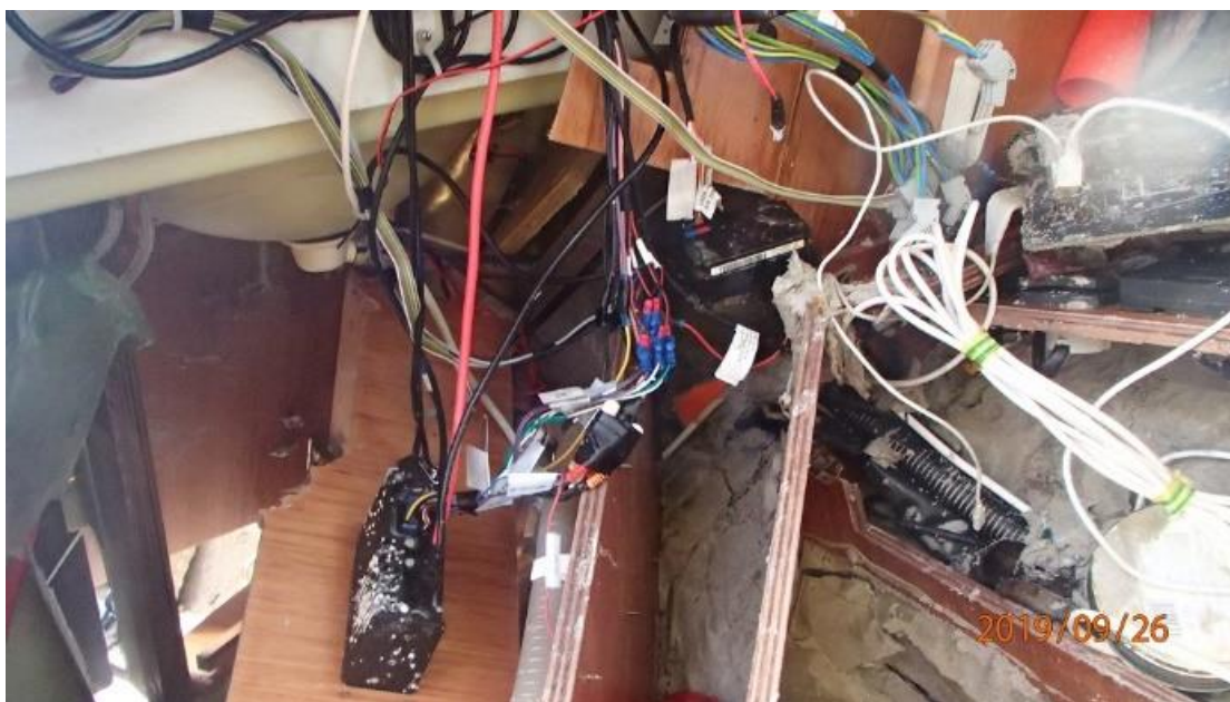
Photograph 13. Radio and navigation station after the accident.
