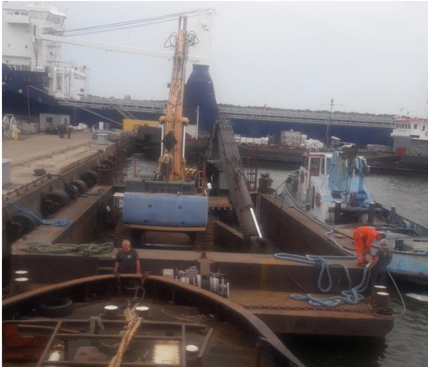
Photograph 3. Position of the excavators on deck
