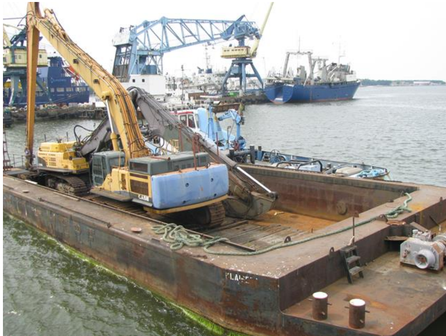
Photograph 2. Position of the excavators on deck
