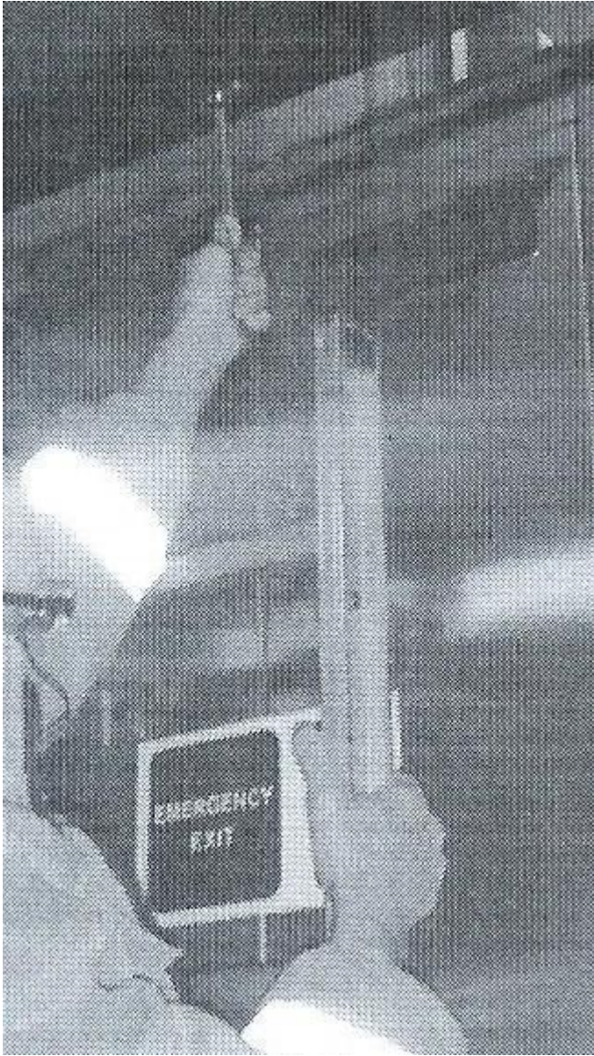
Figure 9. Emergency opening of the hatchway of the lift with the help of special key.
