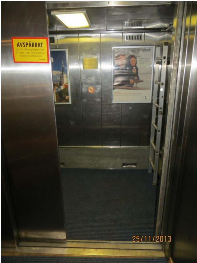
Figure 3. General view of the lift after opening of the door. The ladder of emergency landing from the cabin of the lift can be seen at the right side.
